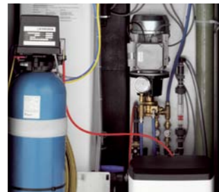
Durable technology Water softening systems prevent lime deposits and guarantee the durability of the system.
